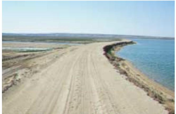
Reinforcement of the dyke with reed faggots
